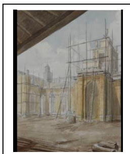
The building under construction
